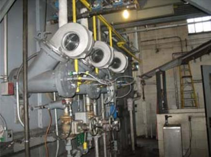
(Image 5.2: Right-Hand View of Burner 2, 4, and 6)
